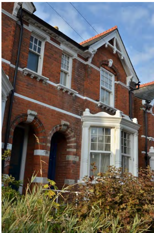
Figure 61, left: note the little white modillions under the eills and the decoration around the inset porches and first floor window arch.
