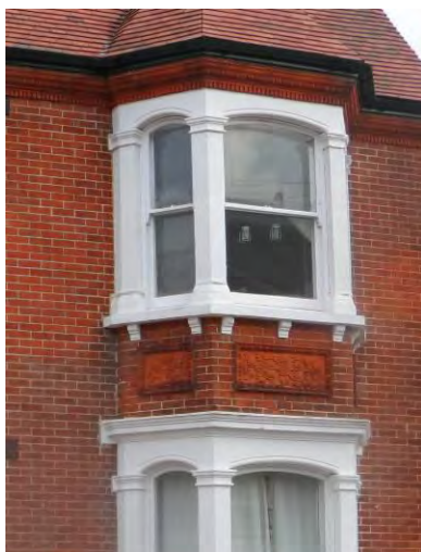
Figure 59, left: Terracotta used at eaves to create the effect of an architrave and on the bay to enrich an area of plain brickwork between ground and first floor windows
