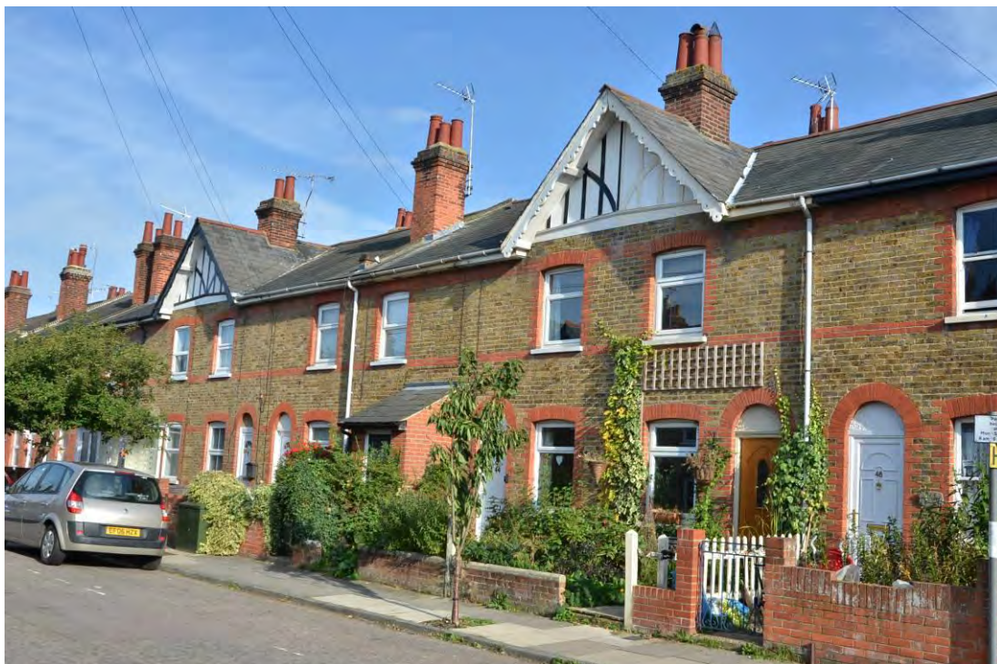
Figure 65: The round-topped doorways echo the inset porches in a more modest way and the red brickwork decorates the yellow London stock bricks simply but effectively. Note the mock half-timbering and decorative fretwork of the bargeboards. The survival of front boundaries and the well-planted gardens define the private spaces despite their diminutive size.
