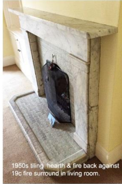
Living room. 19c marble fire surround on original chimney breast. Panel infill to left with modern plaster apse. Modern door to garden room to right. Extended window bay.
