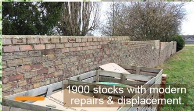
1930/50s picturesque stocks clamp failures
