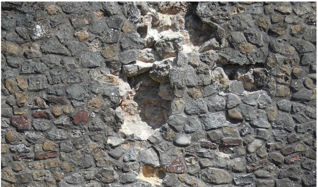
Photograph 2: Repairs in progress at the NW corner of the Town Wall (northern end of Balcerne Hill). Loose septaria and cement mortar (part of the protective skin added during the 1950s and 1960s) have been removed, prior to patching with septaria and lime mortar (May 2017)
