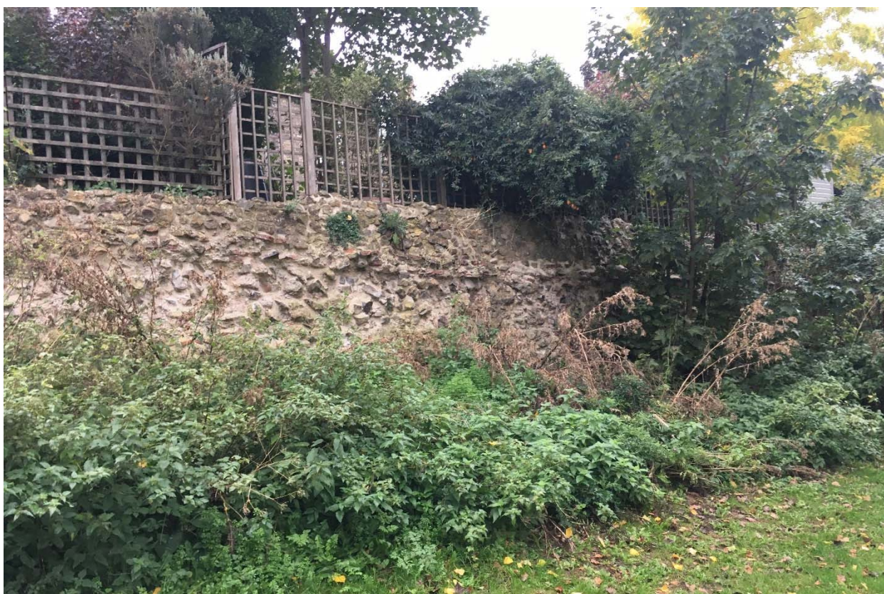
Photograph 13: Vegetation, including a sycamore tree, growing at the base of the Wall. This will cause damage to the Wall and should be removed (October 2018)
