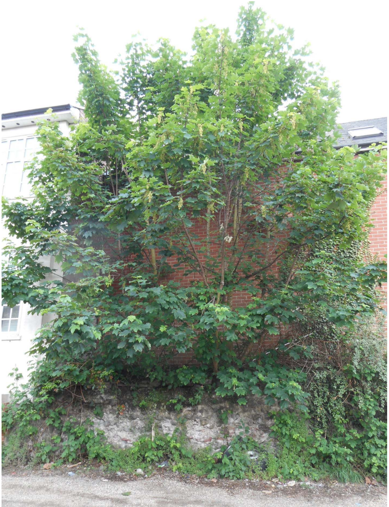
Photograph 11: Sycamore Tree growing on the surviving Wall at St Peter's Street Car Park, prior to removal in 2017. The tree would damage the structure if it was left to grow in this location (May 2017)
