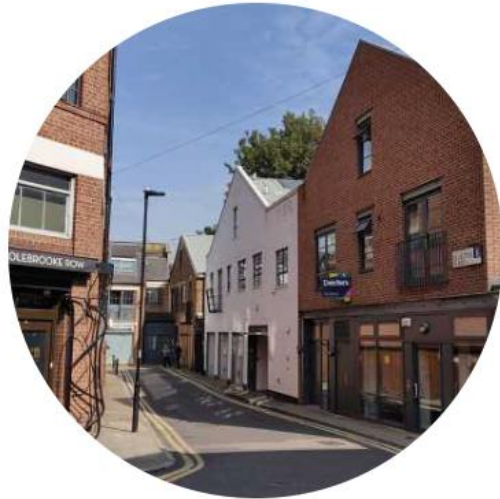
Integration of new with old, active ground floors with residential upper floors - Angel, London
