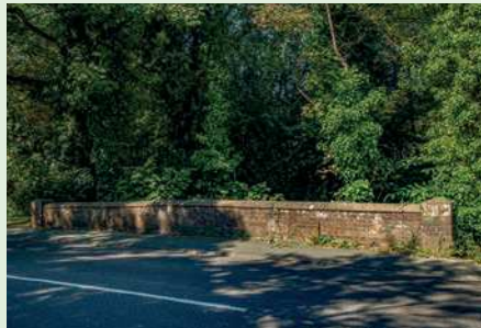
Stanway Bridge, London Road, Copford
