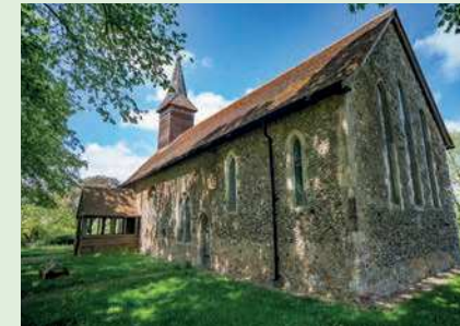
Easthorpe Church, Easthorpe Road, Easthorpe
