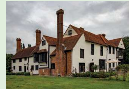
St. Mary's Grange, Easthorpe Road, Easthorpe
