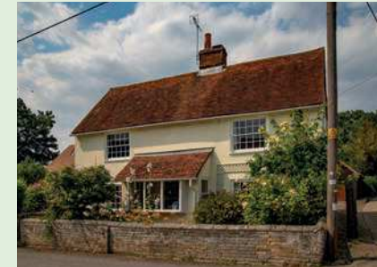
Bell House, Easthorpe Road, Easthorpe
