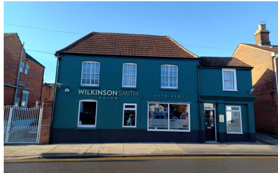
Fig. 70: 66-68 North Station Road.
