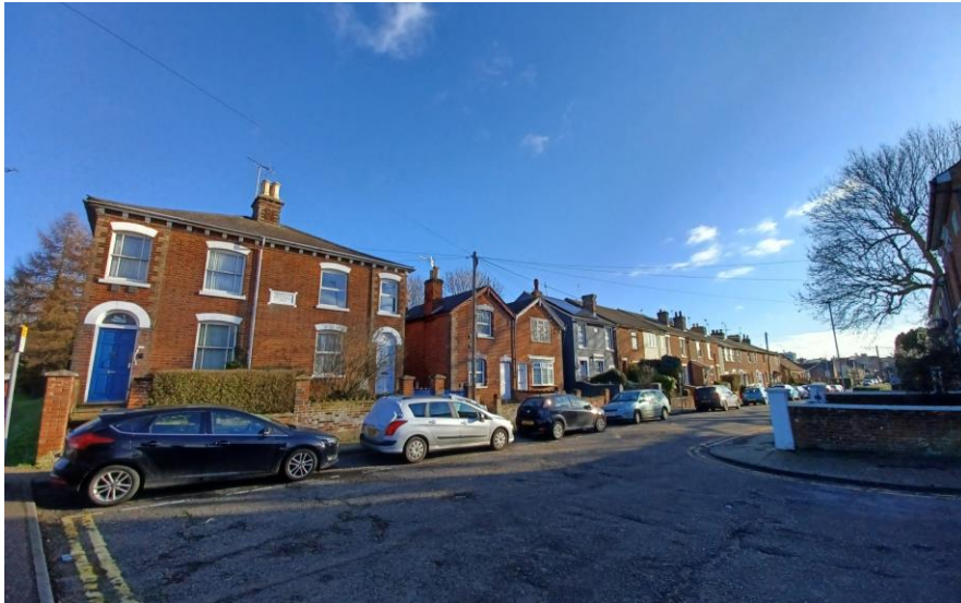
Fig. 81: Belle Vue Road. View from the north end (east side).
