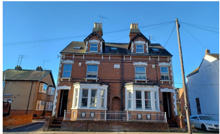
Fig. 71: 60 -62 North Station Road.
