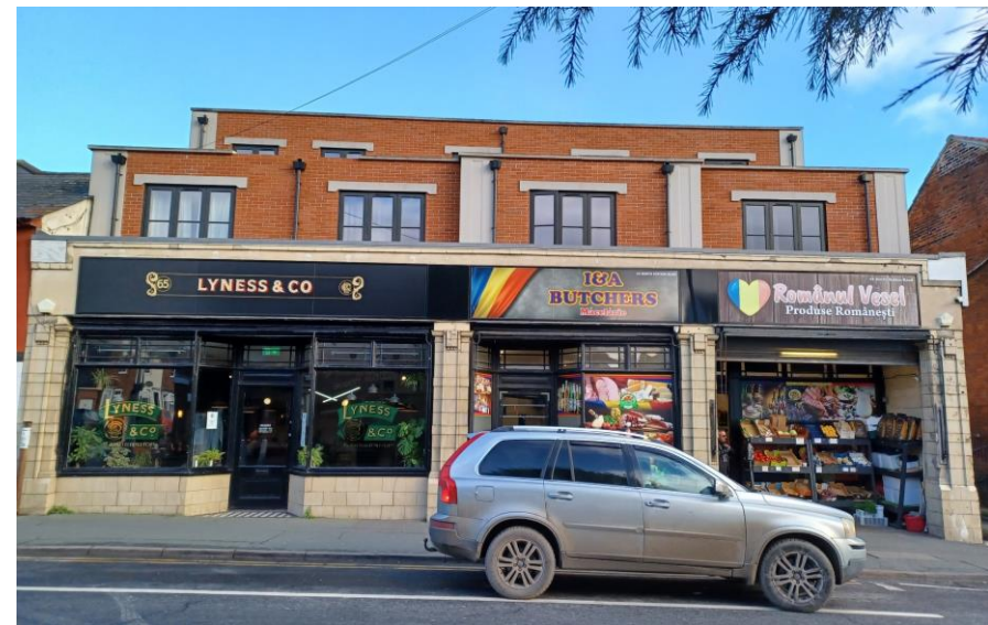
Fig. 63: 63-65 North Station Road.
