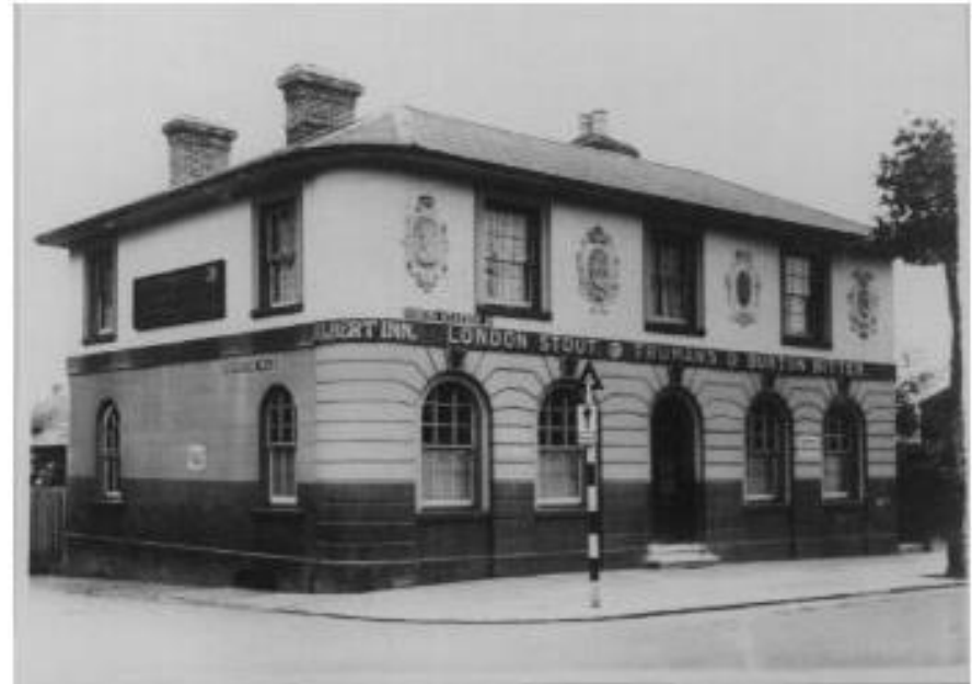
Fig. 50: The Albert Inn, demolished in 1932.
