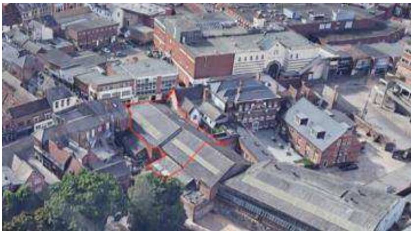
Figure 4: current view of the site from Priory Street (rear), development boundary of scheme highlighted.
