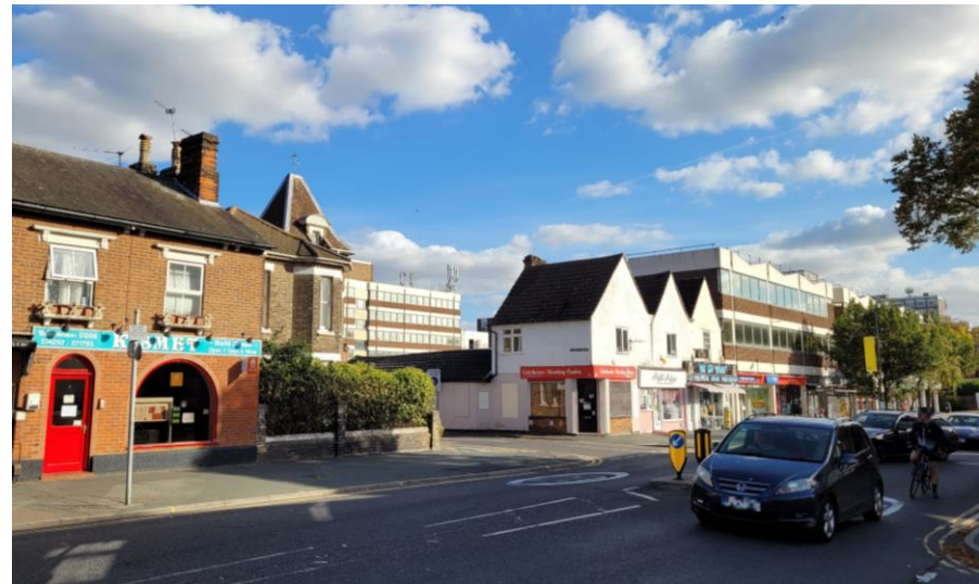
Fig. 58: View of 25-27 North Station Road from the north-west.
