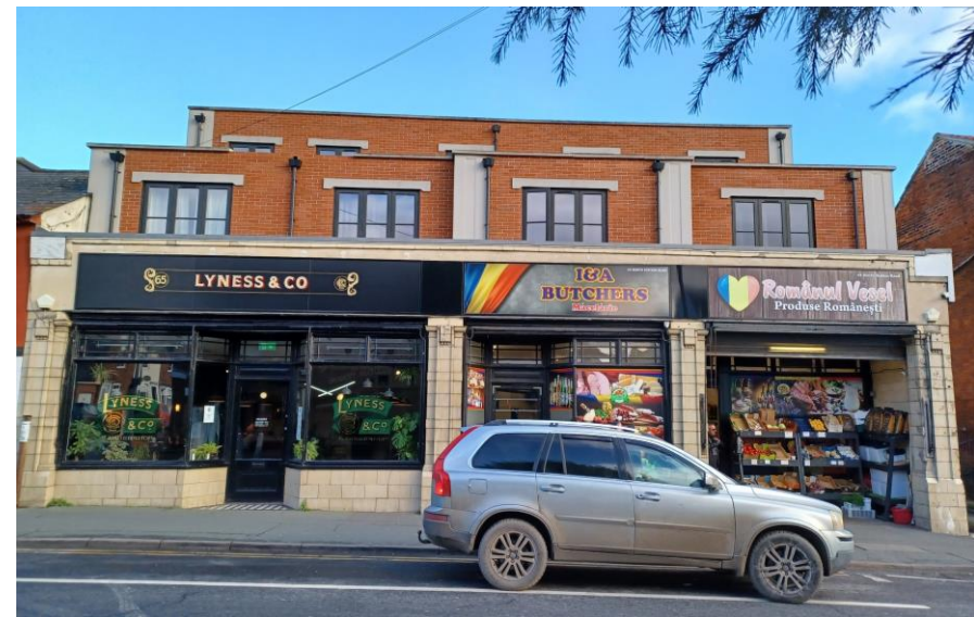
Fig. 63: 63-65 North Station Road.
