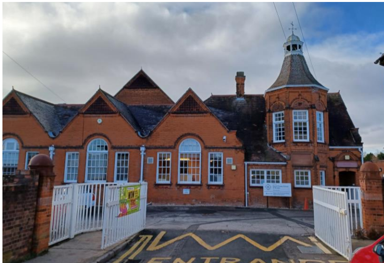
Fig. 23: North Primary School, John Harper Road.
