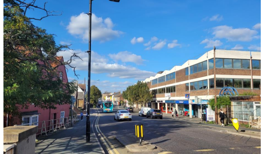
Fig. 57: View of north Station Road from North Bridge with Century House in the foreground.
