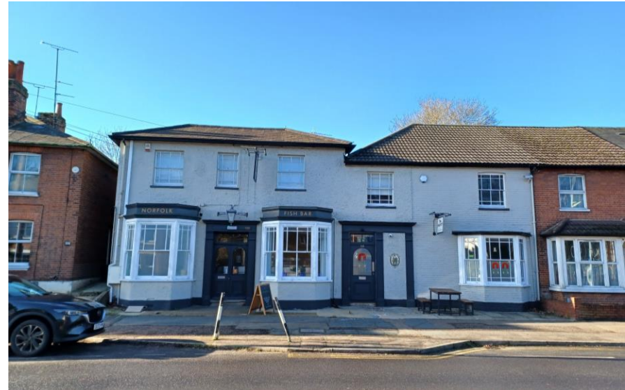
Fig. 80: The Norfolk Pub, North Station Road.
