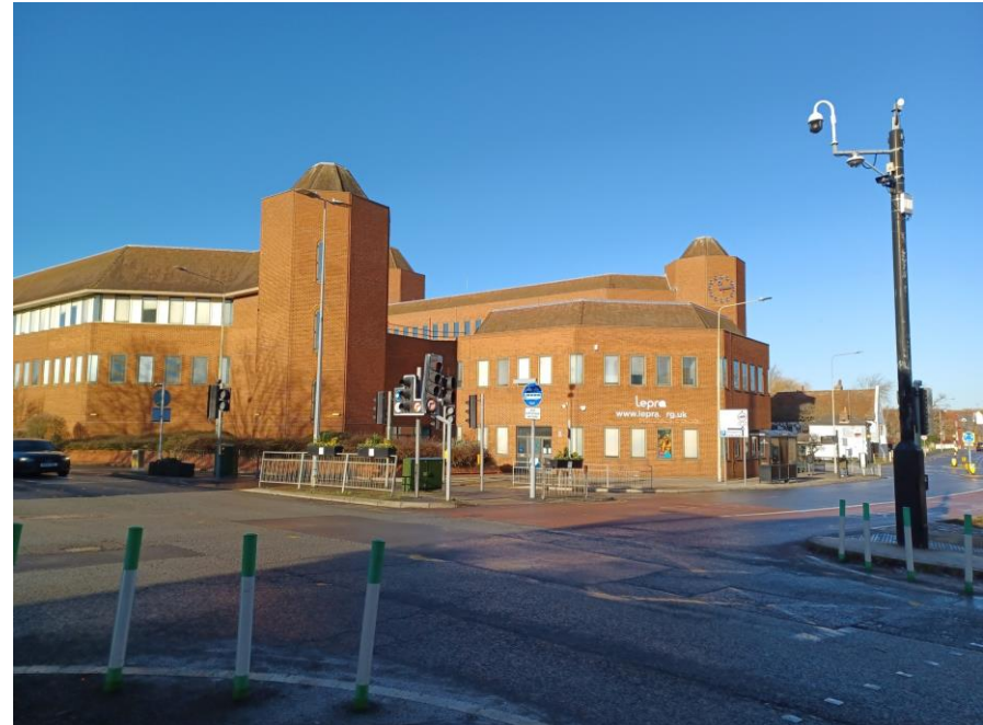
Fig. 47: Pedestrian junction at Middlesborough. View from south-east.
