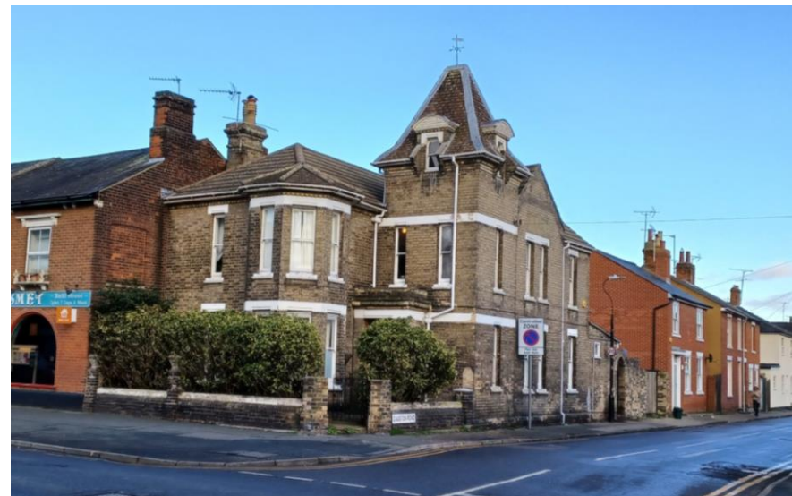
Fig. 60: 29 North Station Road. View from the south-west.
