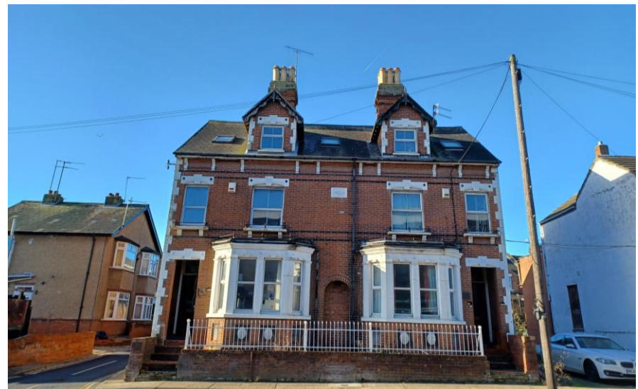
Fig. 71: 60 -62 North Station Road.
