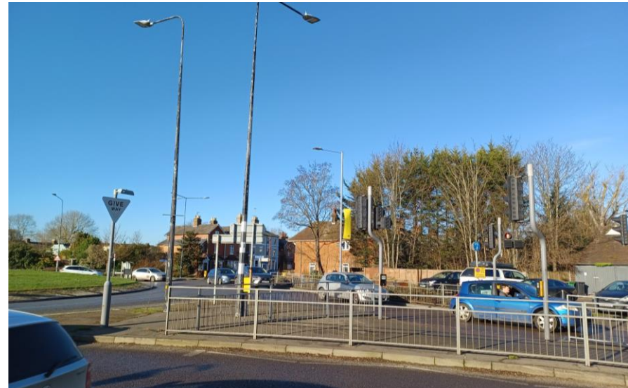
Fig. 72: Pedestrian crossing on the Albert Roundabout.
