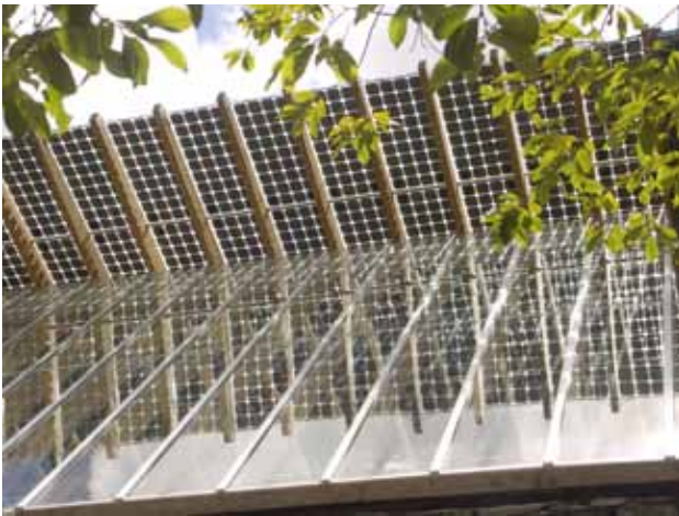
Opportunity for solar panels
