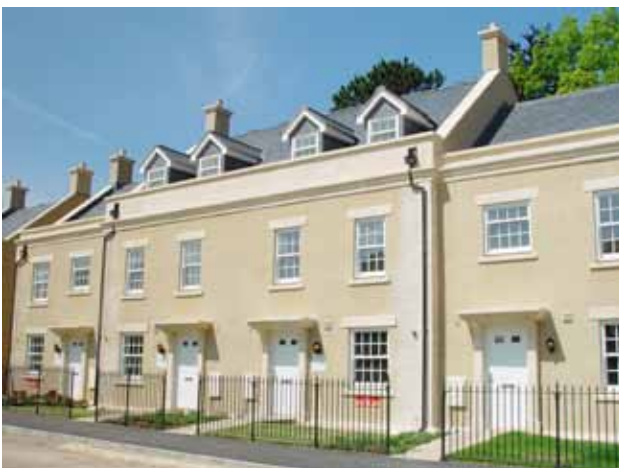
Housing in terraced form
