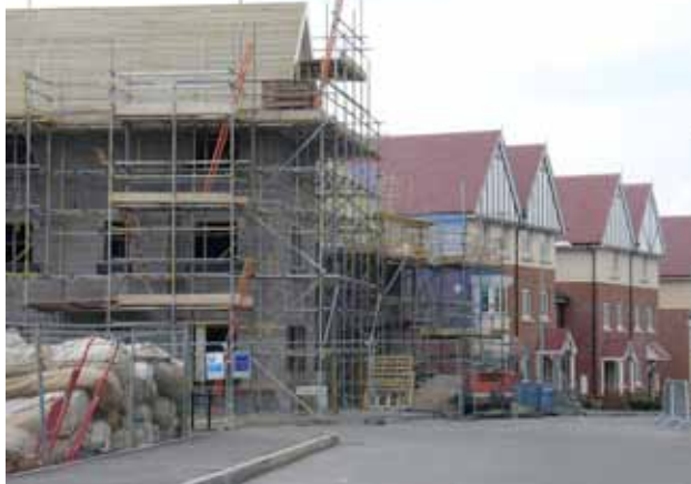
New Braiswick Park under construction
