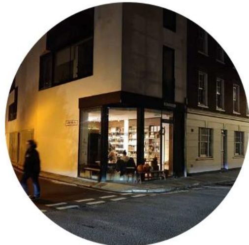
Active corner in a new build within a historic urban fabric adding life to an evening on the street - Bermondsey, London
