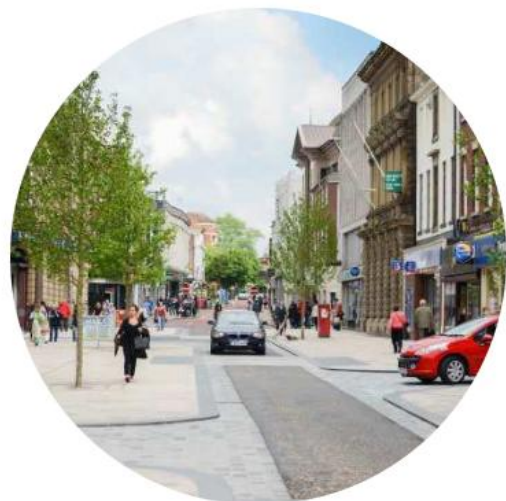
Narrowed carriageways and improved pedestrian environment on high street - Fishergate, Preston
