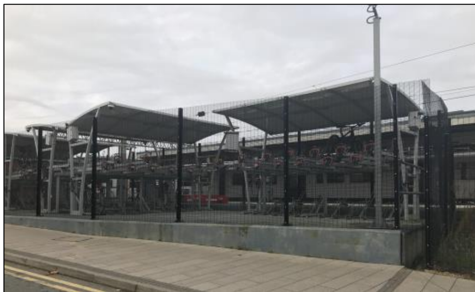
Cycle Parking Compound at Colchester Station
