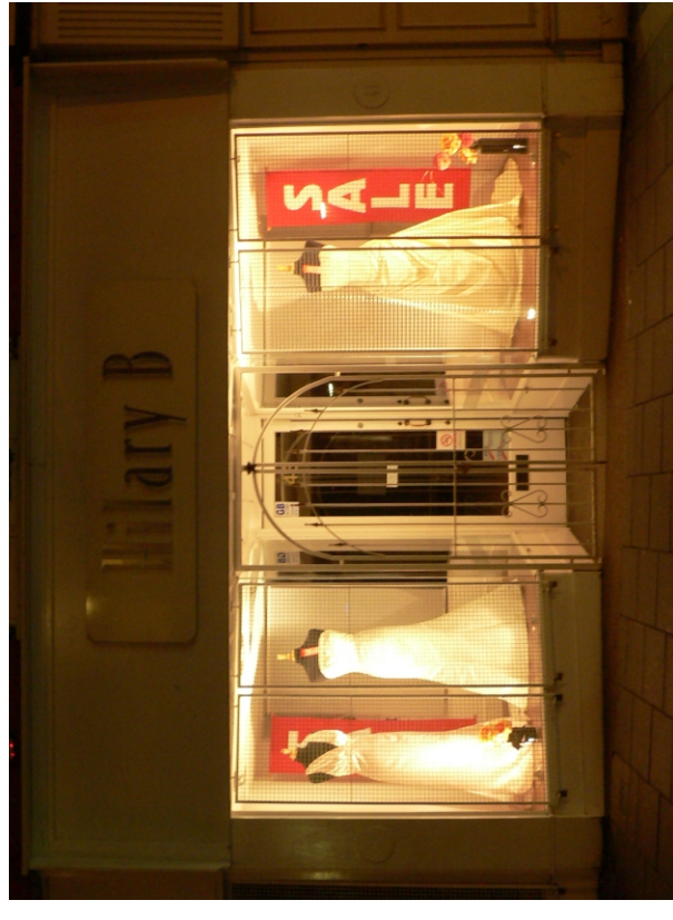
Well integrated de-mountable external grille
