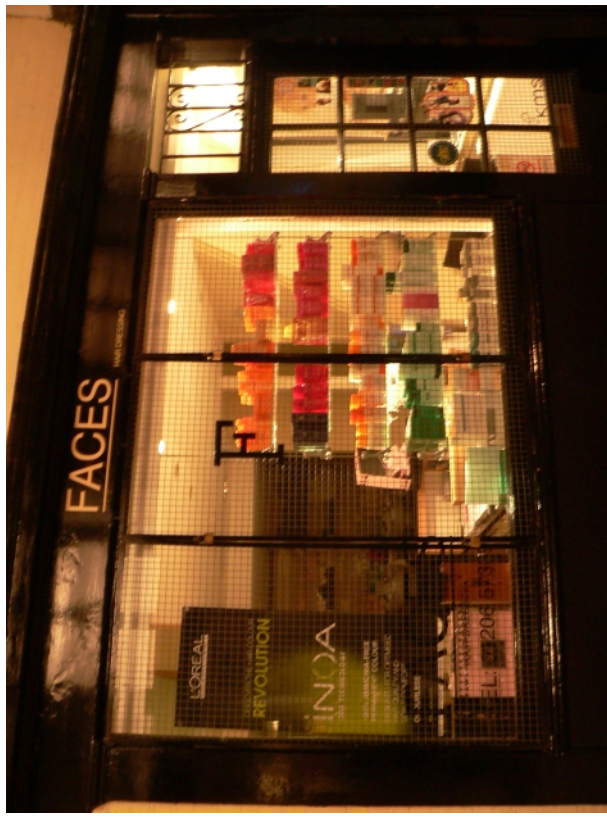
Well integrated de-mountable external grille
