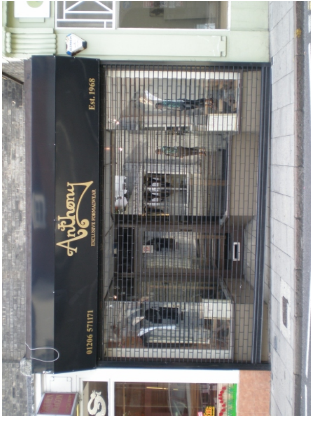
External grille used for enclosure of curved shopfront
