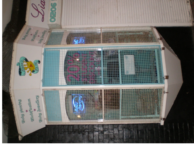
Well integrated grille on curved window
