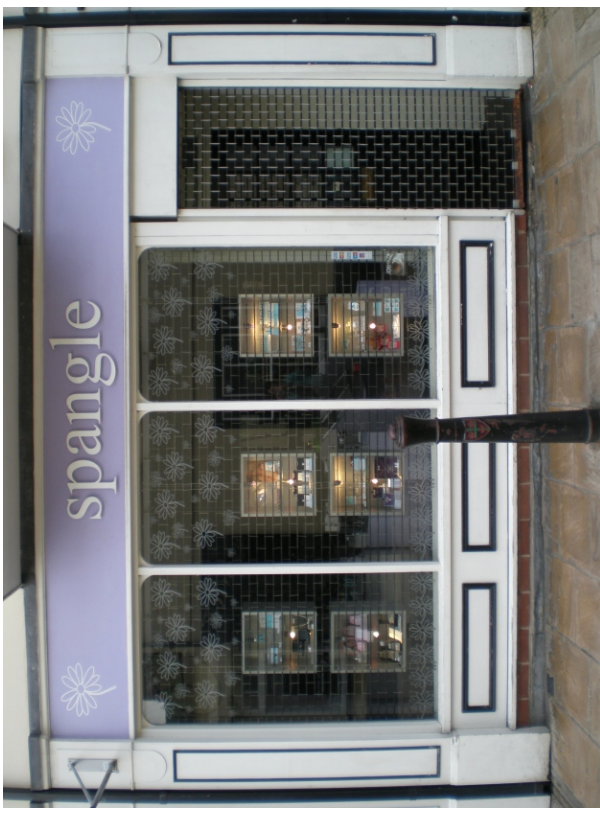
Inconspicuous brick bond internal grille
