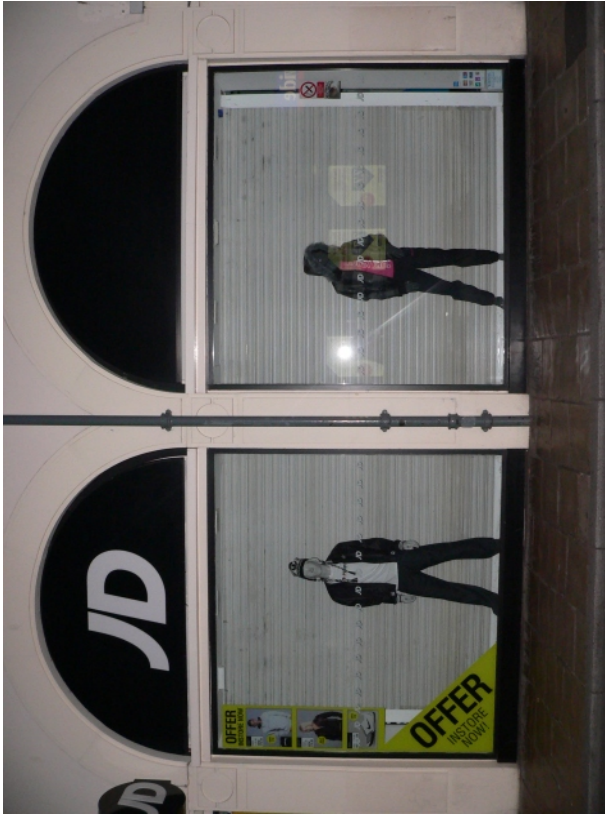
Well integrated internal roller shutters behind display area
