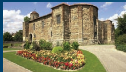
Replacement of heating system at Colchester Castle – estimated saving 18 tonnes CO 2
