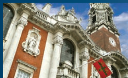
Draught sealing of Colchester Town Hall windows – estimated saving 23 tonnes CO 2
