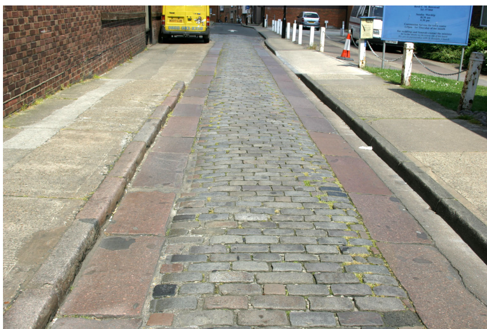
The small section of historic surfacing of the High Street showing the large granite runs for carriage wheels.
