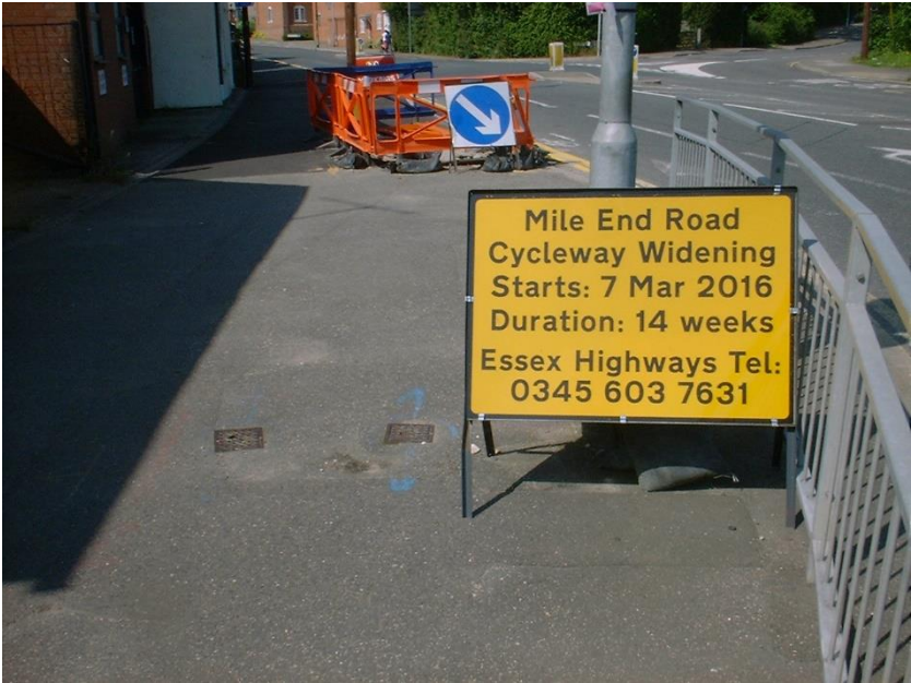
'Work commencing' signage
