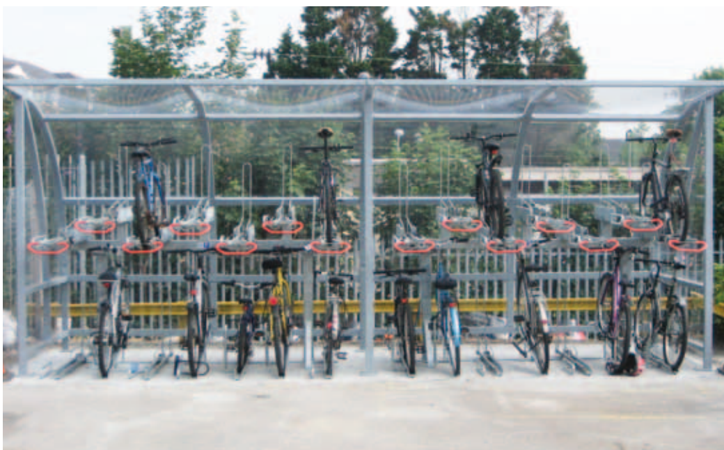
Two tier racks within covered cycle shelter
