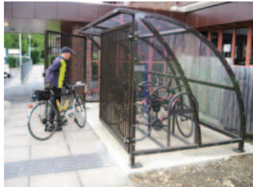
Covered shelter secured with lockable gates
