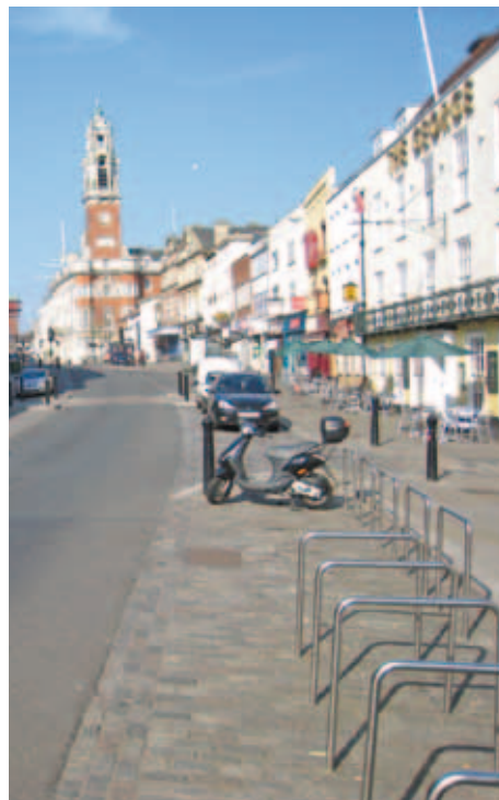
Short term PTW parking, note inappropriate cobbles and manhole cover within parking area
