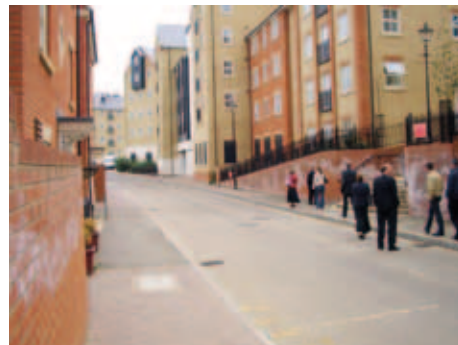
No on-street parking due to developer restrictions (site incomplete)
