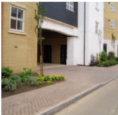
Undercroft secure parking (gated entry).
