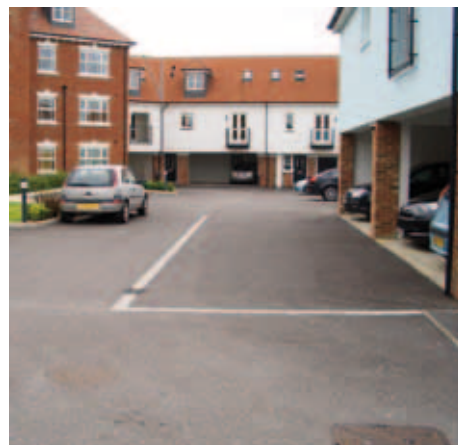
Visible undercroft parking
