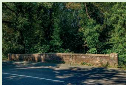
Stanway Bridge, London Road, Copford
