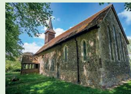
Easthorpe Church, Easthorpe Road, Easthorpe
