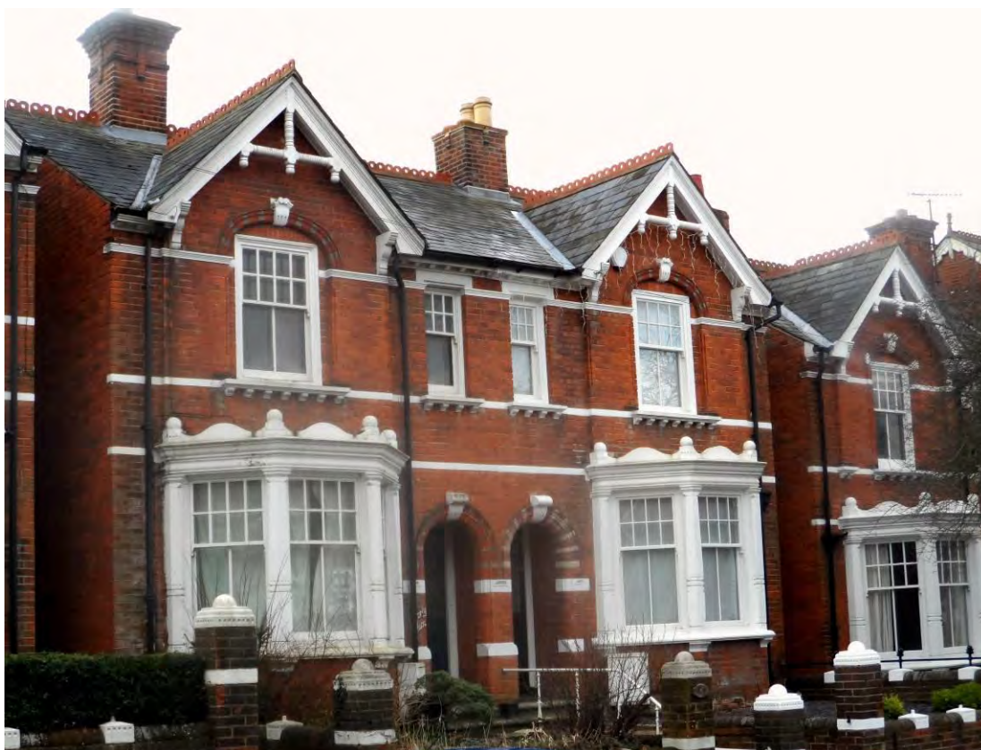
Figure 25: An example of architectural exuberance derived from the combination of polychrome brickwork around windows and doors; white painted enrichment at eaves, gables, string courses, cills, windows and boundary walls; varied roof forms; large elegant bay windows, inset porches and the use of traditional scale and materials.
