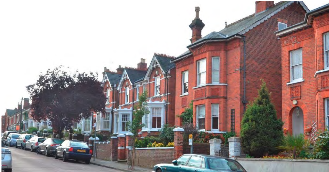
Figure 56: Decorative features can include terracotta lozenges, fretwork on eaves and verges, bays and chimneys
