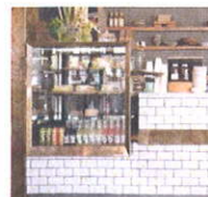
Perimeter display cabinet set into end of bar. Large toughened safety glass display unit with metallic trim to perimeter edges. Internal glass shelving.
