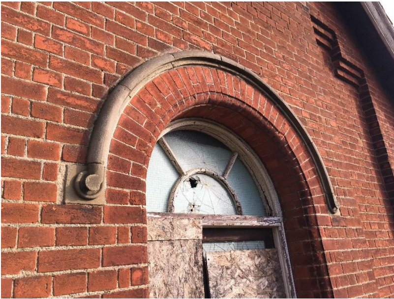
Fig. 3 Detail of stone hood and fanlight above door.
