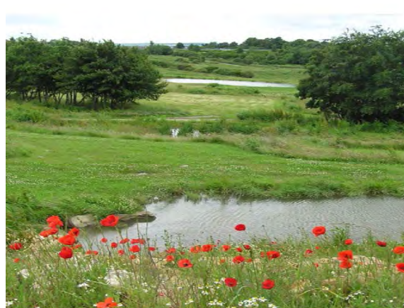
Basins and swales carved from the slopes at Manor Park in Sheffield store and treat run-off from residential areas (above) and are used for events space when dry (below) (Sheffield City Council, 2011)
