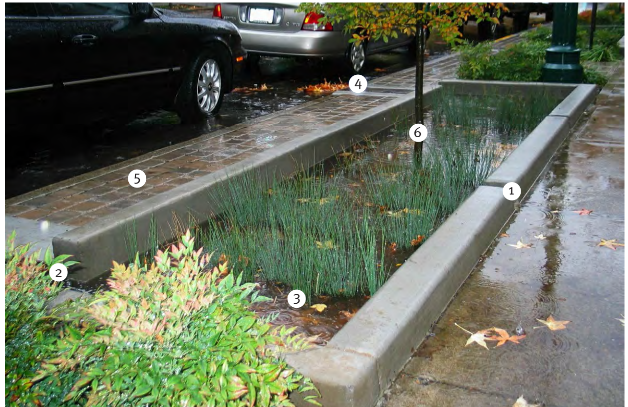
Bioretention planter in Portland
