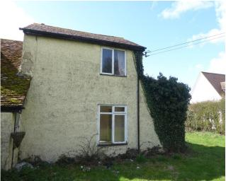
The central section of the property has timber frame walls with a double pitched roof clad with hand made clay peg tiles. There is no information as to the age of this section but I would consider it likely to date back to the late C17th. As will be seen; very little of the original fabric remains.
