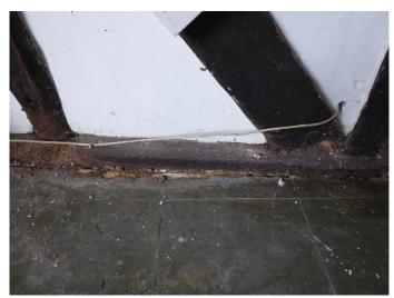
The first floor is suspended timber. Floor joist ends are supported by perimeter walls and by a large central beam spanning between walls. The original floorboards have been replaced with modern tongue and groove with no historical value.
